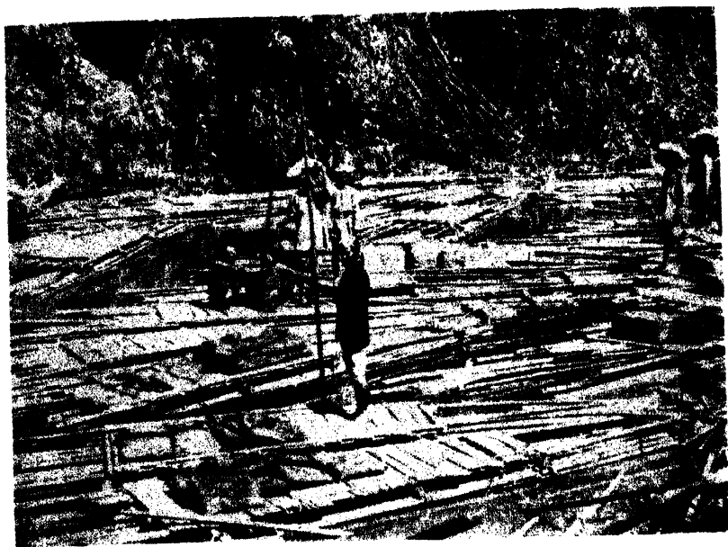
RAFTS ON THE KLONG RIVER BEING LOADED FOR THE NORTHERN COLUMN.
